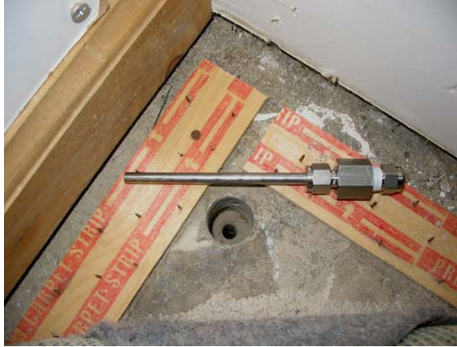
Assembled subslab port ready for installation
